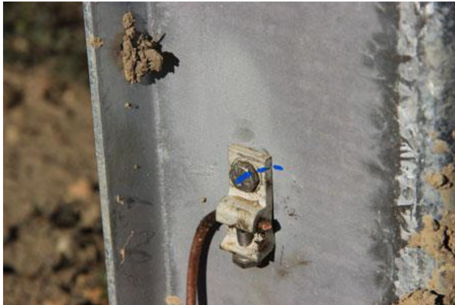
Figure 2. Bonding washers in conjunction with hold-down clamps and bolted joints (Smalley, 2015)
